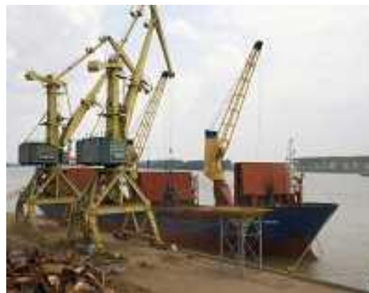
Figure 12: Cranes installed at the port of Galati.
