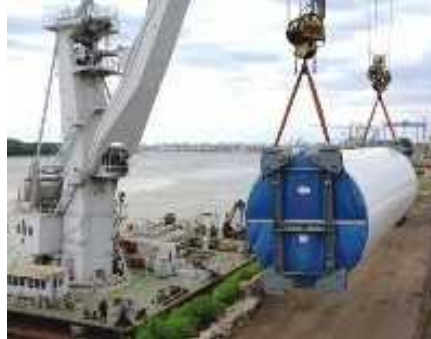
Figure 13: Self-propelled crane installed at the port of Galati.
