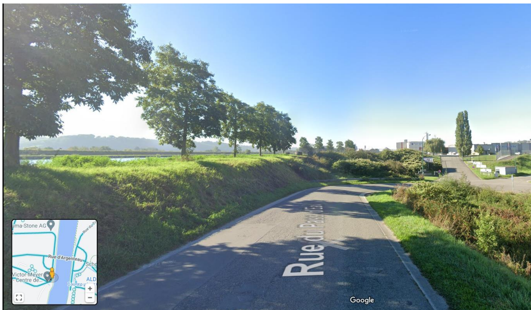
(c) West dike
